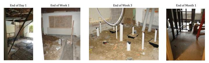
By June 20<sup>th</sup>, the construction permit was in place and the *initial* inspections for the framing, electrical, plumbing, and HVAC had been completed. The restroom framing and drywall were being installed, and the air conditioning units were being hung throughout the house as well as the ceiling tiles and LED lighting.
