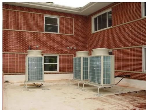
The rooftop air conditioning units were dropped in by crane and set in place as shown to the left.
