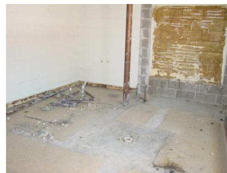
3rd floor restroom above
